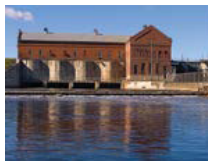
Grand River Webber Dam In-service: 1907 Capacity: 3.225 MW
