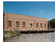
Kalamazoo River Calkins Bridge Dam In-service: 1936 Capacity: 2.55 MW
